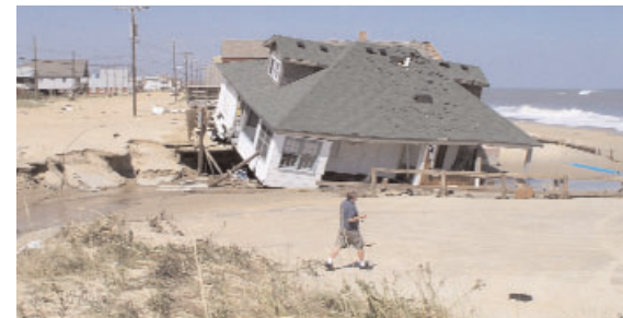
Damage caused by Hurricane Isabel at Kitty Hawk, N.C.
