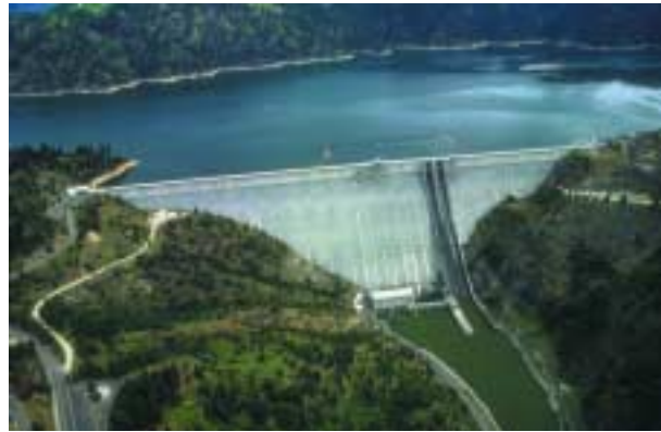
Aerial view of the Dworshak Dam on the North Fork of the Clearwater River in northern Idaho.
