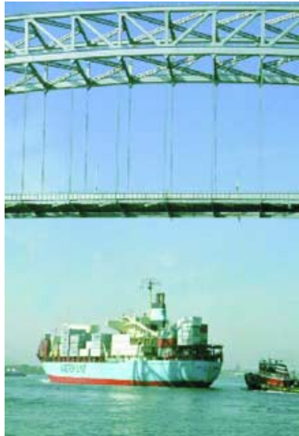
A container vessel navigates the Kill Van Kull channel as it passes under the Bayonne Bridge, New Jersey. The Corps has deepened this channel to accommodate modern shipping vessels.
