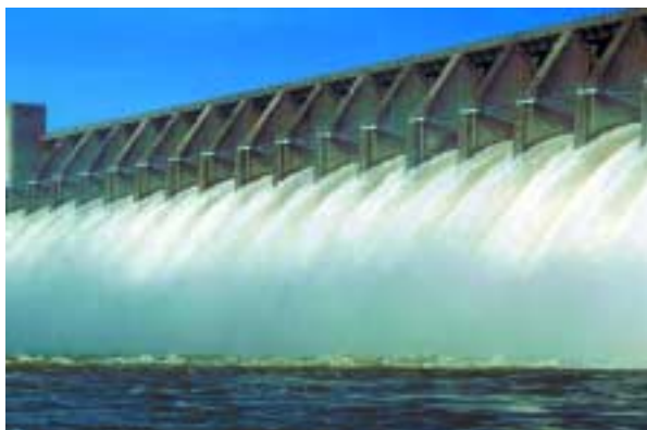
J. Strom Thurmond Dam and Lake, Flood Gates, Clarks Hill, South Carolina.
