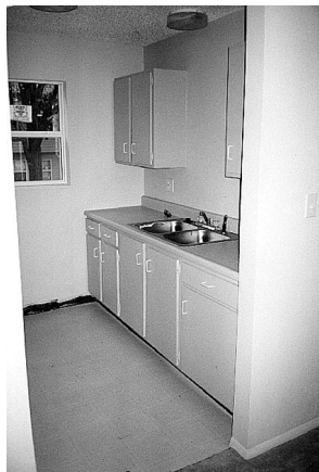
Newly renovated kitchen
