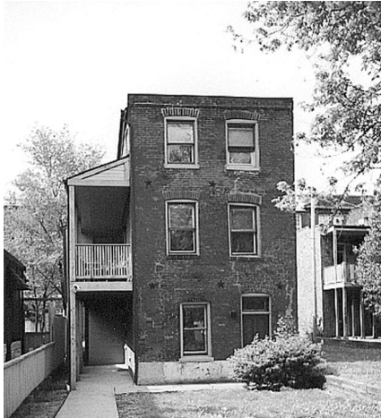
Renovated -unit town house, previously fire damaged
