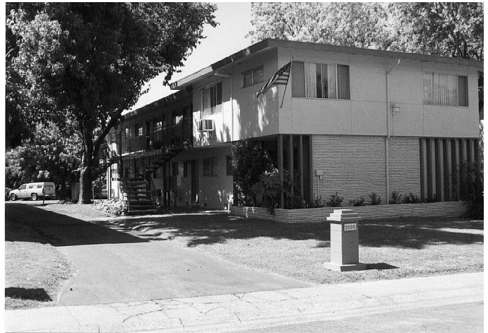
Neighboring property recently purchased by new owner
