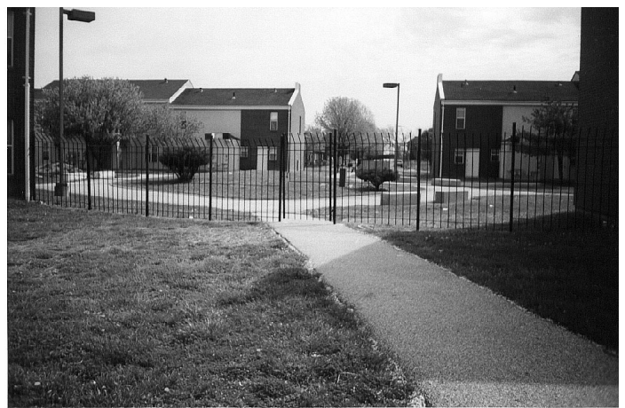
New wrought iron security fence and lighting
