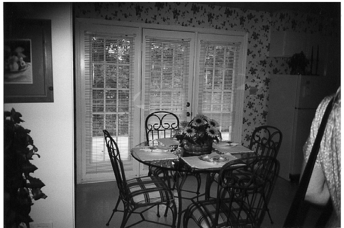
rench doors replaced sliding glass doors
