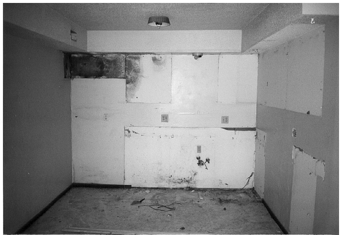
uninhabitable unit undergoing gut rehabilitation
