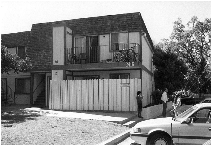
New roof, gutters, and painting
