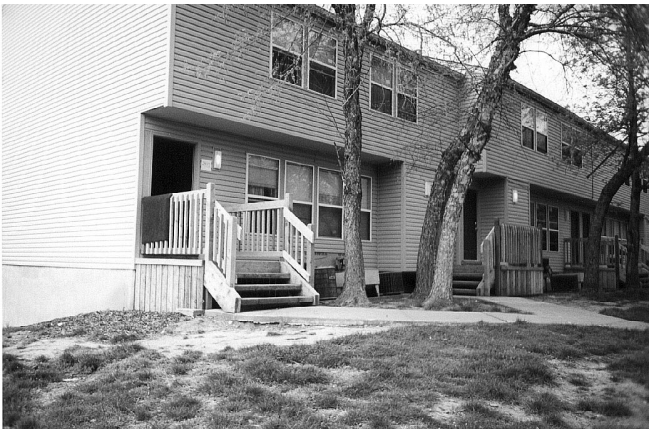
New vinyl siding windows, and steps
