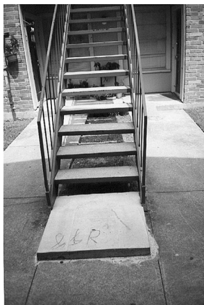
Repaired balcony steps
