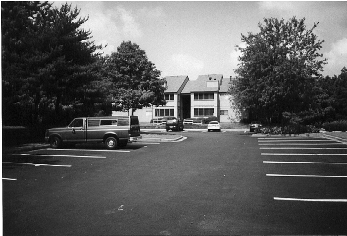
Repairs to interior roads and parking area
