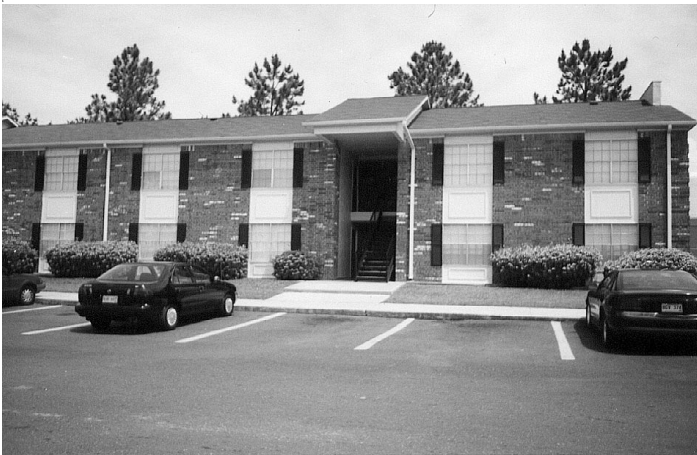
Typical building, new roof, gutters, painting
