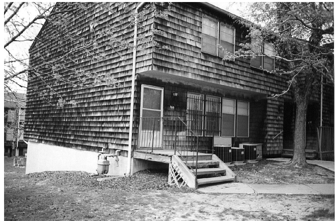
isting wood siding windows, and steps
