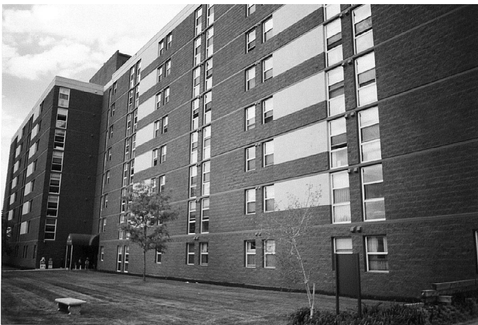
Subsidized units for the elderly/disabled in a high-rise building
