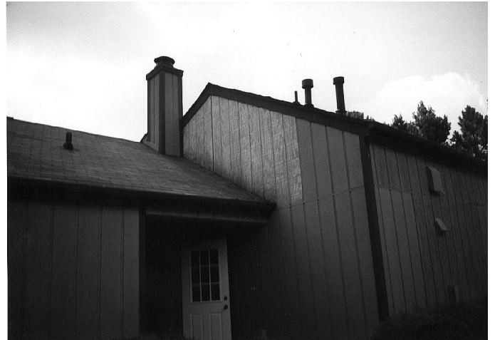
Water-damaged siding replaced
