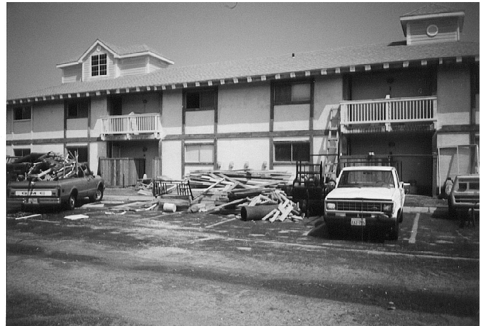
reparation of exterior for painting
