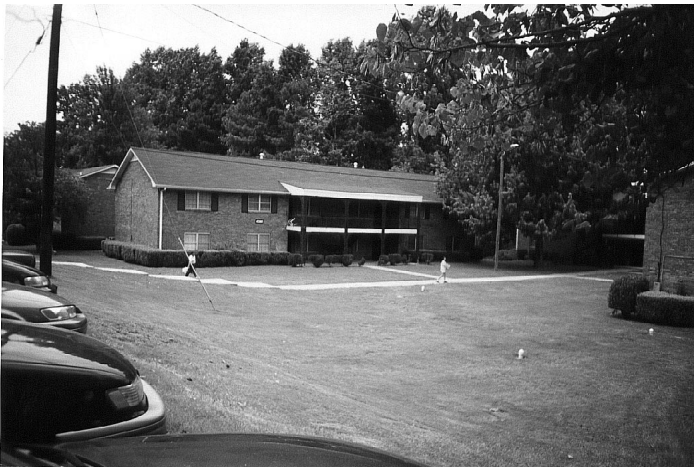
New roof, gutters, and landscaping
