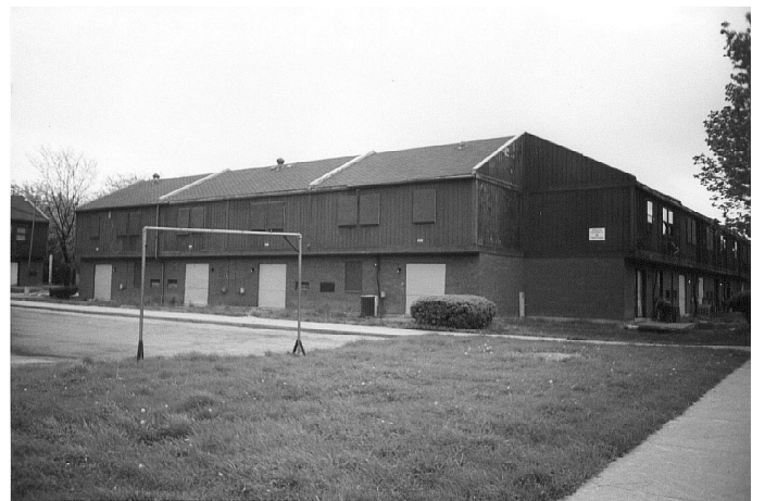
Boarded-up units in adjacent Murphy Blair Townhouses
