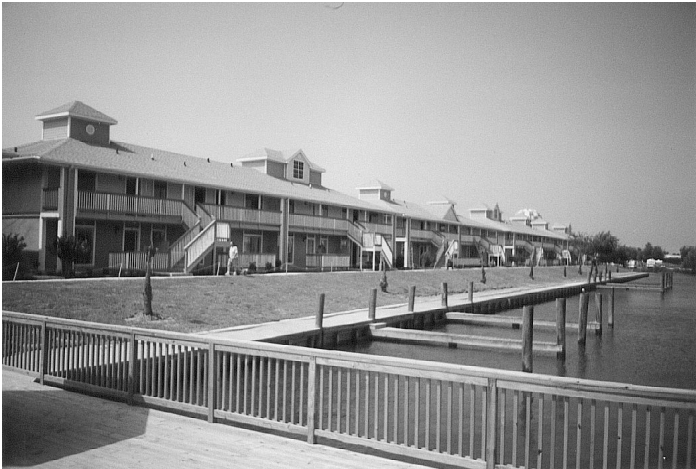
New roof, balconies, and steps
