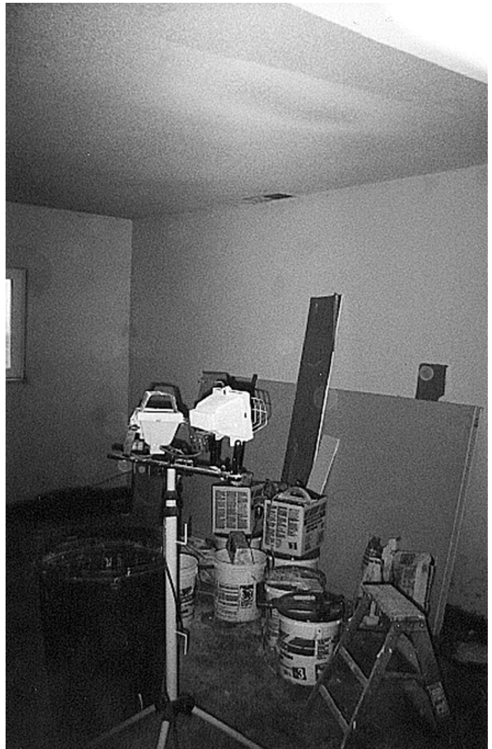
Gutted unit undergoing rehabilitation
