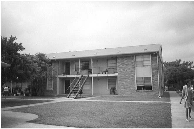
New roof, gutters, painting, landscaping
