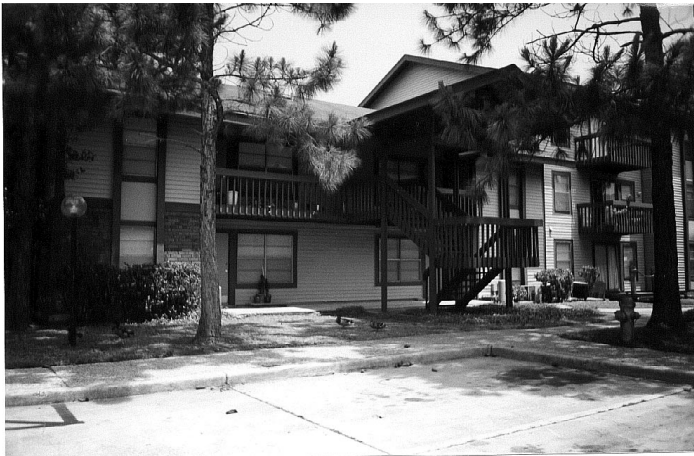
New vinyl siding and freshly painted wood trim
