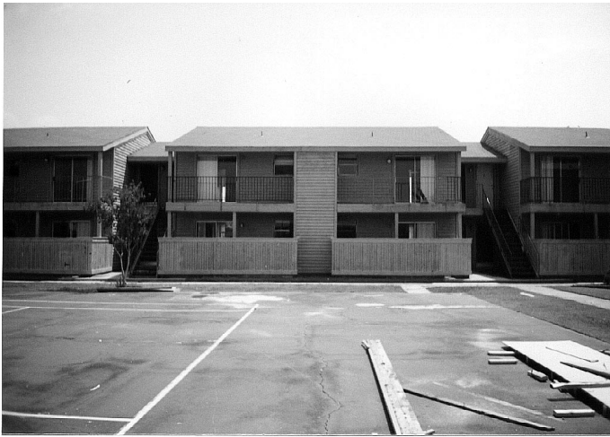
Typical building with new roof and gutters
