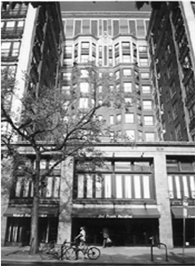
Building, commercial space on first two floors, top two floors closed off
