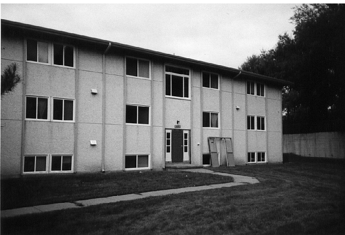
Replacement of entrance door and side window panels
