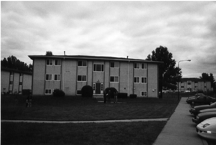
New roof, windows, and exterior painting
